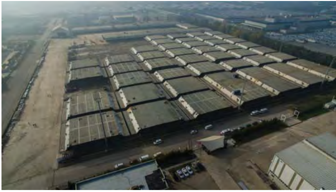
Site Assembly and storage of Deck
